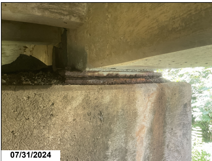
Span # 2, bent # 2, girder # 2: active corrosion with pack rust.
