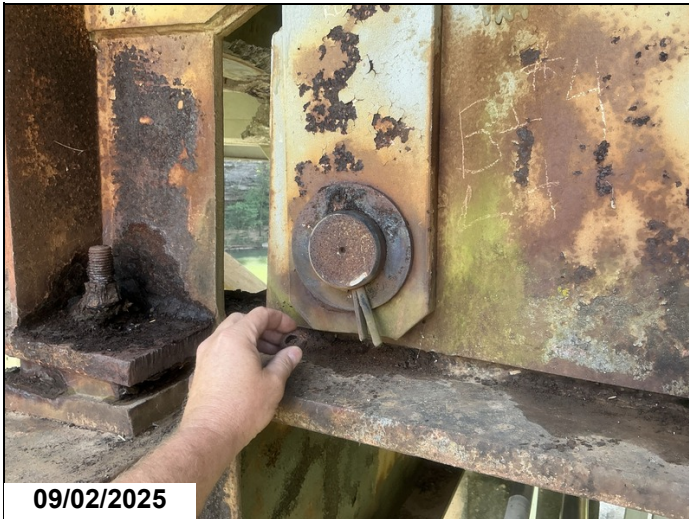
Bent # 4, span # 3, left: pin hanger assembly with fractured cotter pin.
