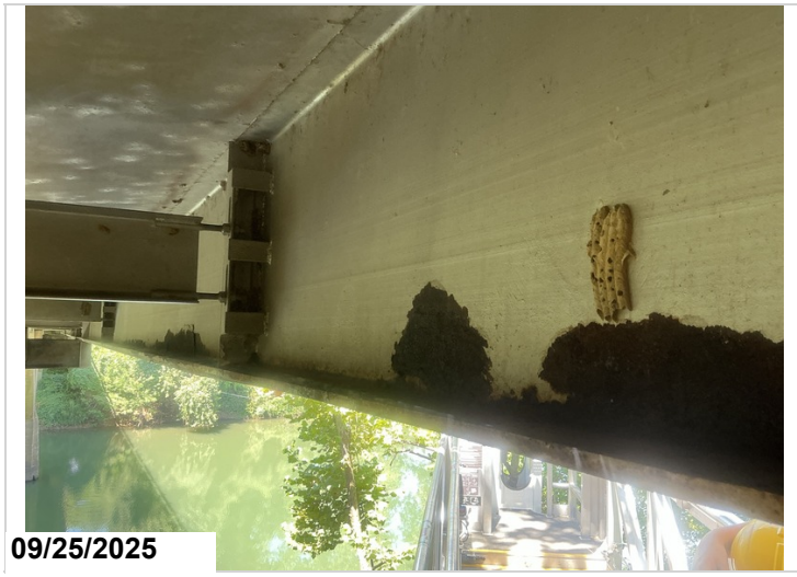
The girders have a failing paint system.
