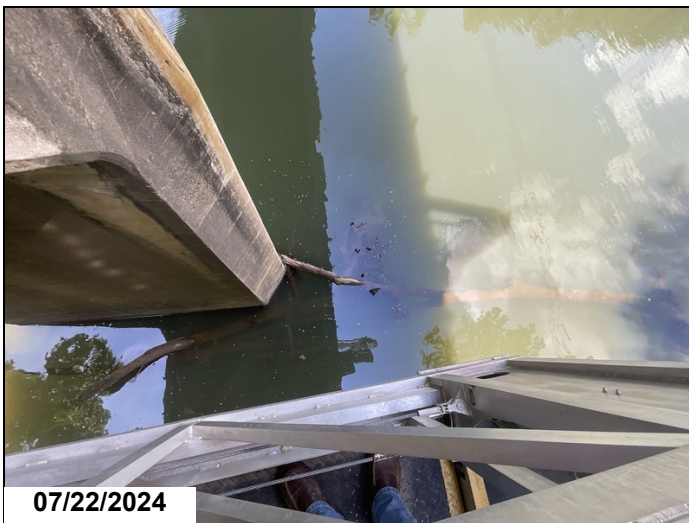
Submerged drift accumulation at bent # 5.
