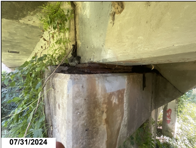
Bent # 2, girder # 5: bearing has active corrosion and pack rust.
