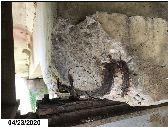
Span # 2, girder # 1-Spalling with exposed reinforcing steel.
