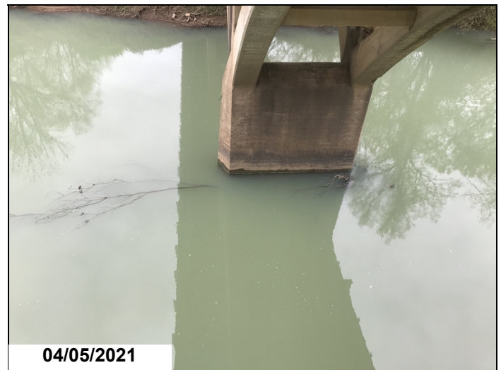
Submerged drift accumulation at bent # 5.
