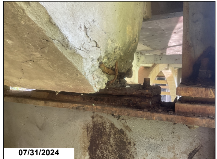
Span # 2, Bent # 3, girder # 5: bearing has active corrosion and pack rust.
