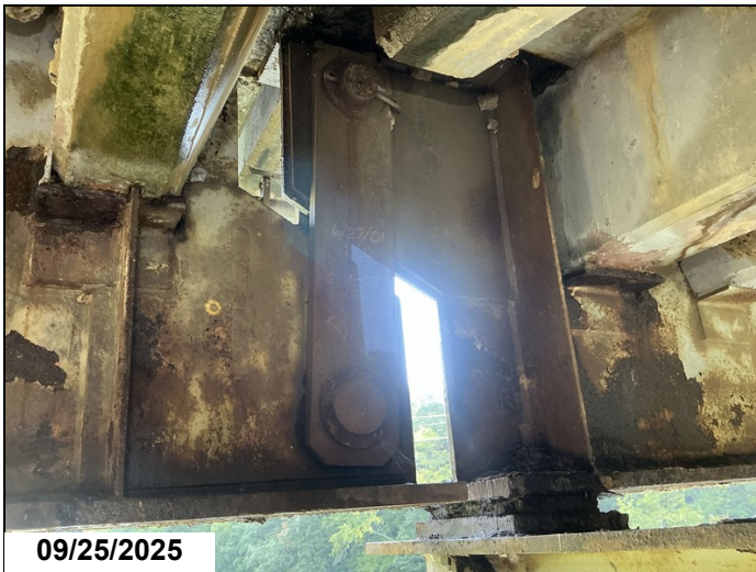
Pin hanger assembly, bent # 4, girder # 1: typical.
