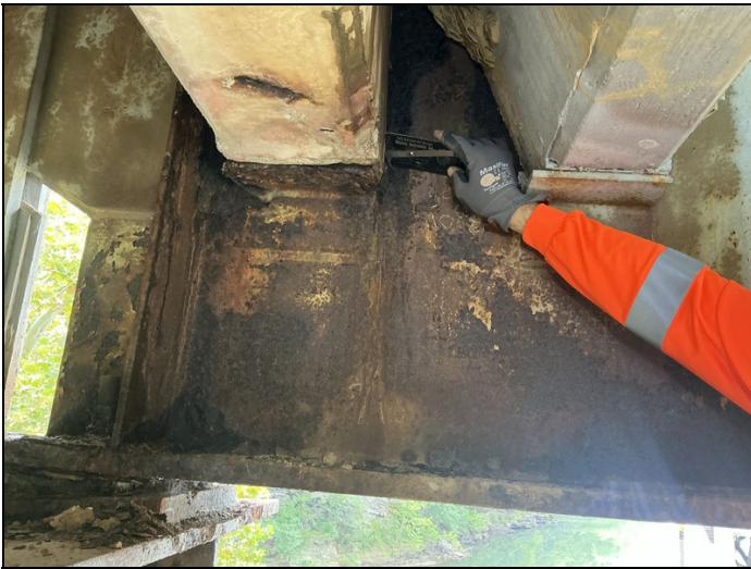
The girder ends and bearings have active corrosion and pack rust.
