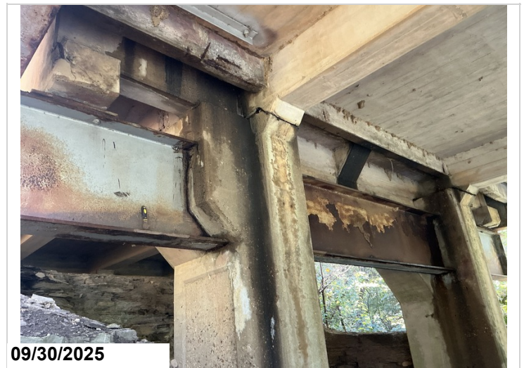
NSTM Steel Bent Caps.
