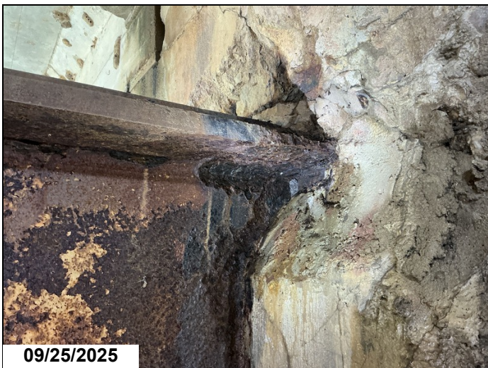
Bent # 5 Steel Cap, Center section between the columns: The steel cap section between the concrete columns has active corrosion, flaking rust and section loss up to 1/4" on the web adjacent to the top flanges at the column juncture. The top flange has up to 1/2" section loss along the edge of the flange.
