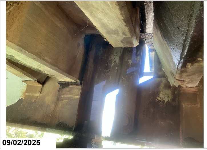
Bent # 5, Span # 5, girder # 1: pin hanger assembly.
