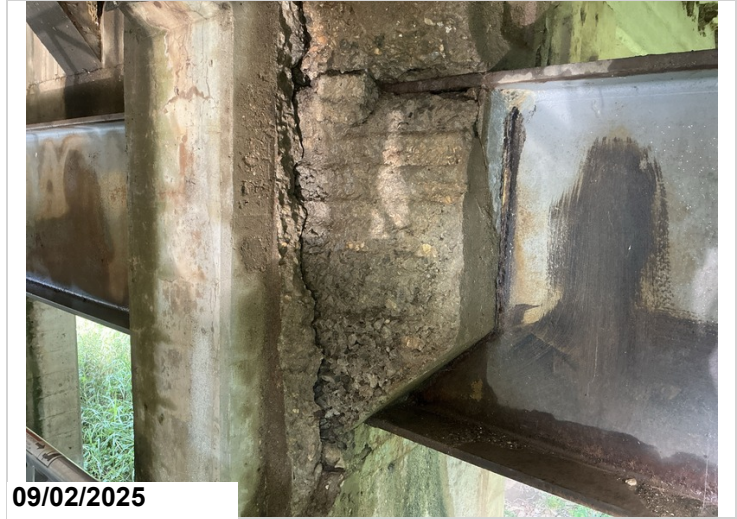
Bent # 3 ahead face. The top of the left column of bent # 3 has vertical and diagonal cracking approximately 3/8" wide with a delaminated area under the bearing for left concrete girder. (This deficiency appears to be similar to the area repaired in the past by installing a vertical support at bent # 5, column # 1 as noted above.)
