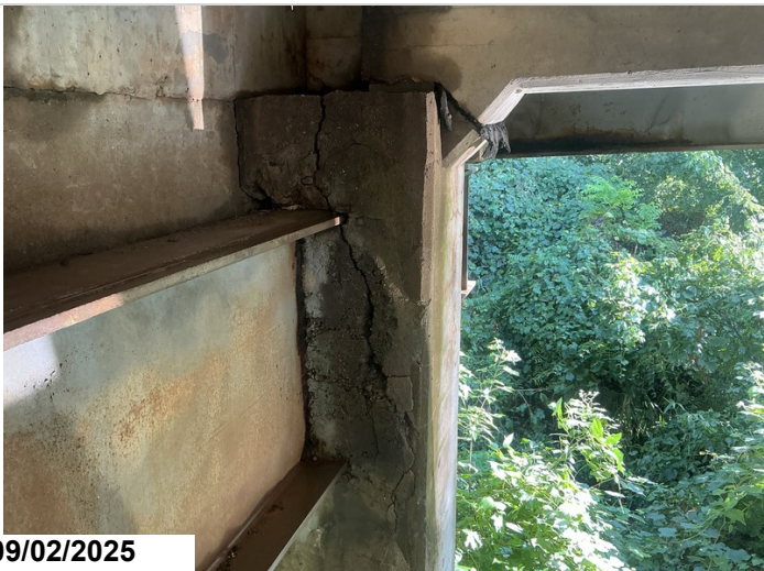
Bent # 3 ahead face. The top of the left column of bent # 3 has vertical and diagonal cracking approximately 3/8" wide with a delaminated area under the bearing for left concrete girder. (This deficiency appears to be similar to the area repaired in the past by installing a vertical support at bent # 5, column # 1 as noted above.)
