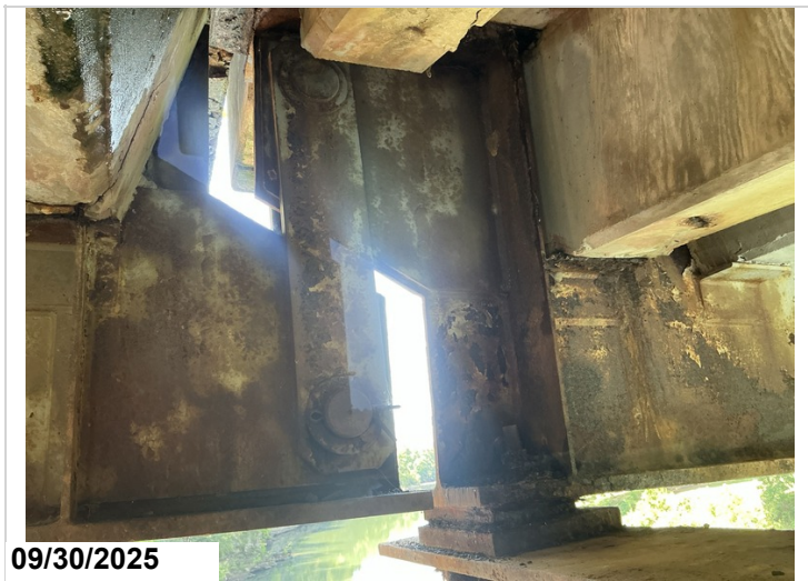
NSTM Pin Hanger Assemblies.
