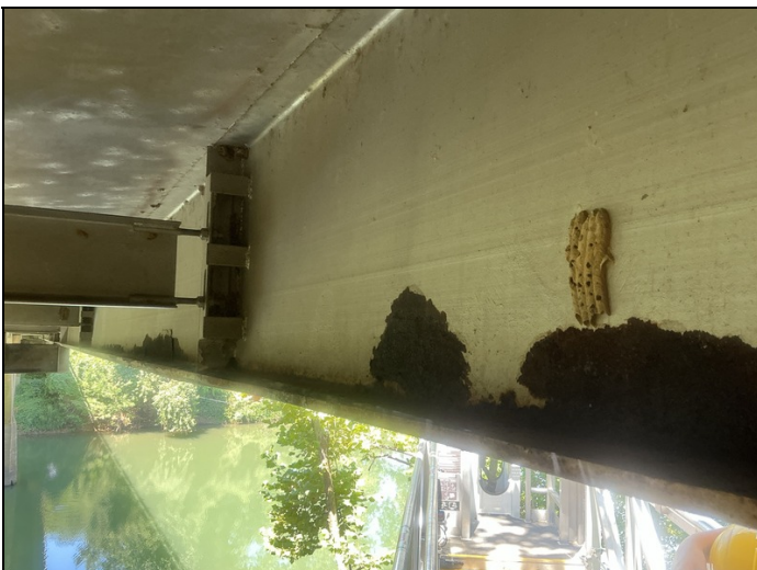
The girders have a failing paint system.
