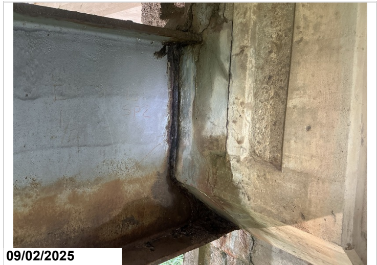
Bent # 3 Steel Cap, Left side: The Span # 2 side of web has 5/16" section loss to the steel cap at the juncture where the w-beam passes through the (original) reinforced concrete cap.
