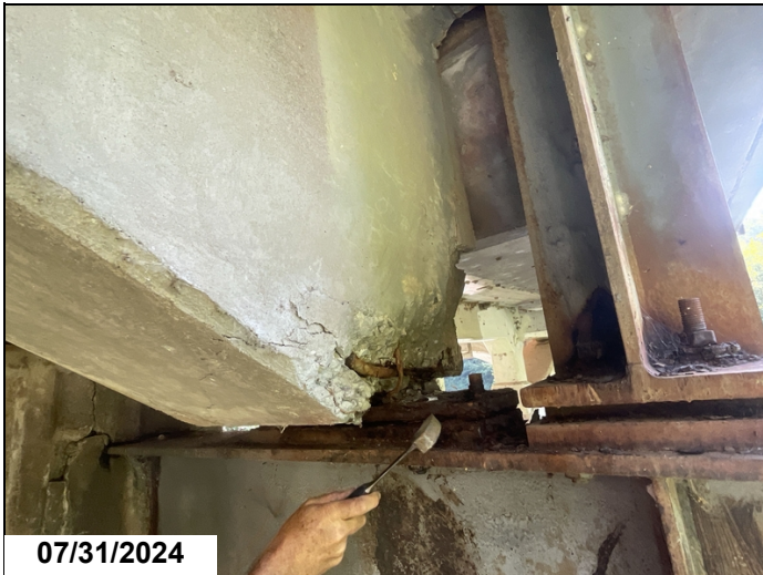
Span # 2, bent # 3, girder # 5: concrete spalling with exposed reinforcing steel, exposed reinforcing steel has up to 75% section loss.
