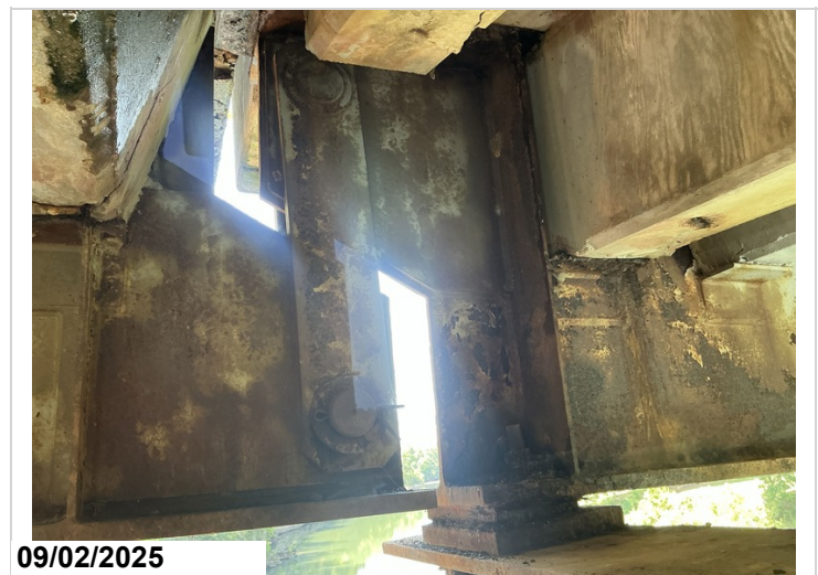
Pin hanger Assembly, Bent # 5, girder # 4: typical.
