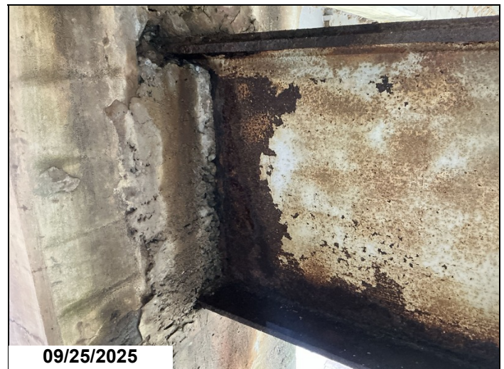
Bent # 4 Steel Cap, Center section column # 2 The steel cap section between the concrete columns has active corrosion, flaking rust and section loss up to 1/4" on the web and top and bottom flanges at the column juncture.
