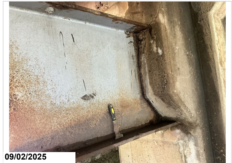
Bent # 6 Steel Cap, Left Side: The Span # 5 side of web has 1/8" section loss to the steel cap at the juncture where the w-beam passes through the (original) reinforced concrete cap.
