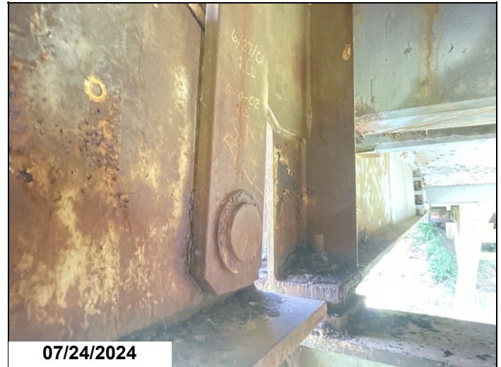
Bent # 4, span # 3, left: pin hanger assembly with active corrosion behind the pin hanger.
