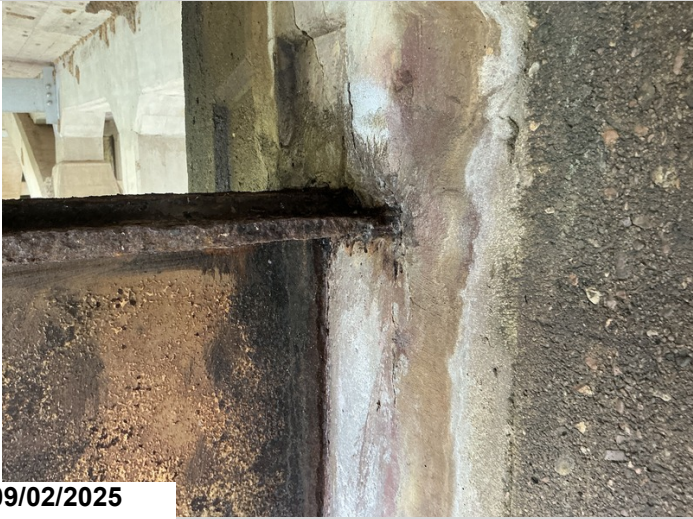
Bent # 5, Span # 4 , left: the top flange has been reduced to 5/16" thickness.
