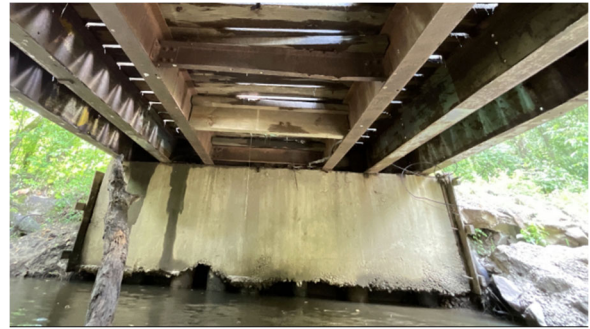
Figure 1 Undermining of the abutment exposing piles.
