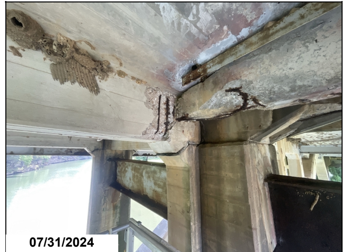
Bent # 4, span # 4, girder # 2, left: spalling with exposed reinforcing steel.
