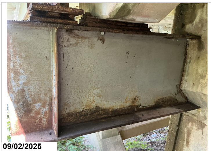
Span # 6 Steel Cap, Right Side: The Span # 5 side of web has 1/16" section loss to the steel cap at the juncture where the w-beam passes through the (original) reinforced concrete cap.
